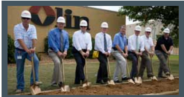
Olin Chlor Alkali Products broke ground Friday, July 22, 2011, on a state-of-the-art membrane cell manufacturing facility at its Charleston plant. The facility is scheduled for completion by the end of 2012. The new plant will have a production capacity of 200,000 tons. It will produce chlorine, caustic soda, potassium hydroxide and related products.
