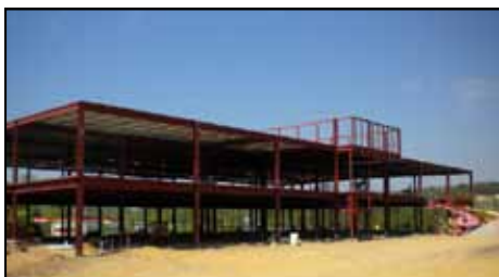
In Progress Photo of 150 Office Park
