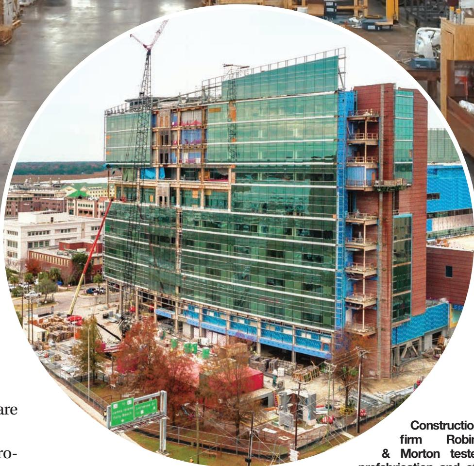
Construction firm Robins & Morton tested prefabrication and off-site manufacturing for the \$256 million Medical University of South Carolina project in Charleston. Much of it was built in an 80,000-square-foot warehouse 15 miles outside the city.
