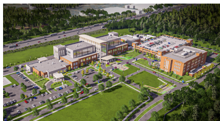
CAROMONT HEALTH CRMC - BELMONT HOSPITAL, MOB AND PARKING DECK BELMONT, NORTH CAROLINA
