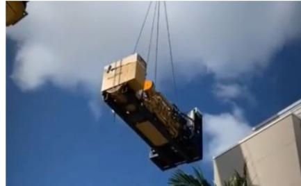
In March, our Joe DiMaggio Children's Hospital project team in Hollywood, Florida, installed a 33,000 pound Caterpillar generator using a 275 ton hydraulic crane in just four hours. This generator will provide a redundant emergency power source for the hospital's existing four-floor facility and the new four-floor expansion set to complete in fall of 2022.
